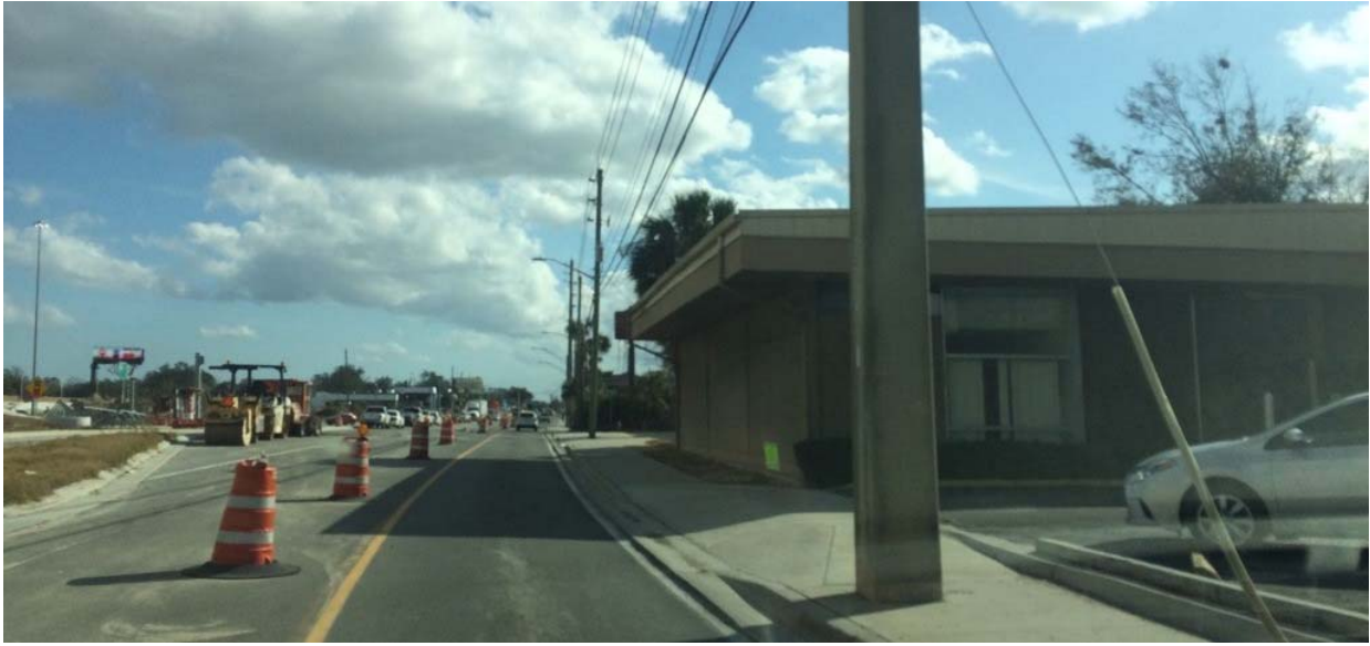
View of the subject property on the right facing south along Kings Ave/Philips Hwy
